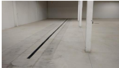
Right: The containment structure minimized contamination during concrete cutting. Above: The completed trench drain.
