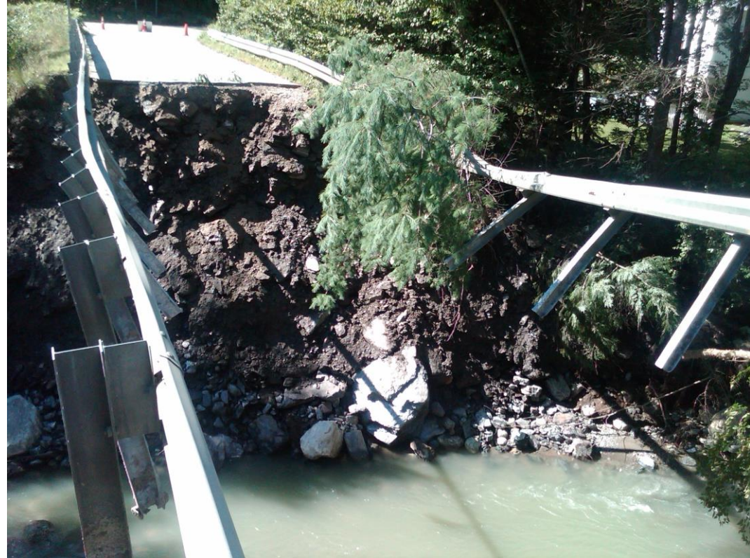
Culvert Failure During Tropical Storm Irene in Townshend, Army Corps of Engineers
