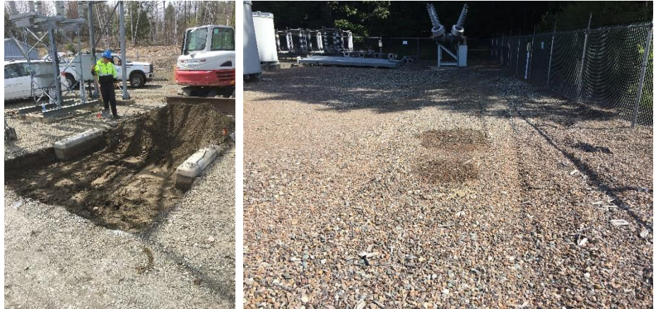
Left: Cleanup of PCB-contaminated soil at the Barre substation. Right: Oil-stained soil identified during a site inspection at the Milton substation.
