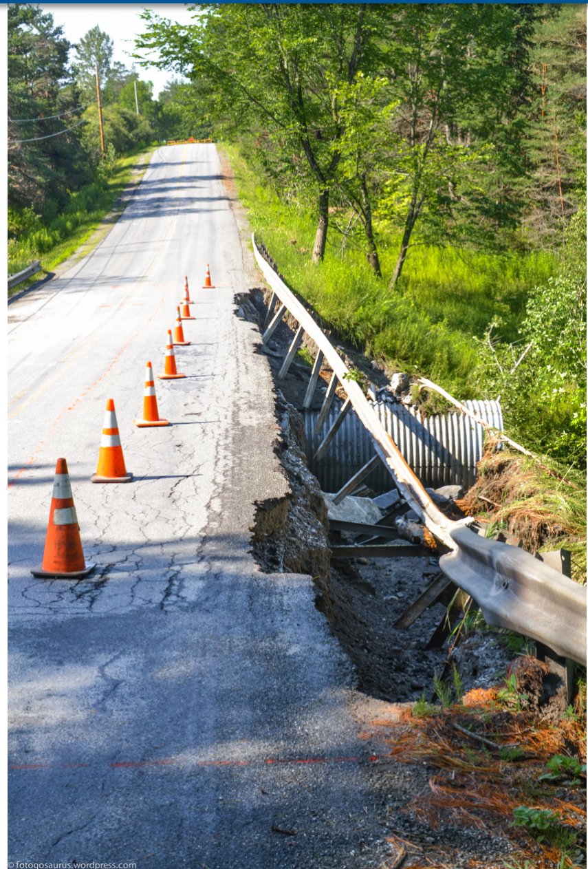
Great Brook Brook Road in Plainfield, VT 7/20/2015 Photo taken by B. Towbin
