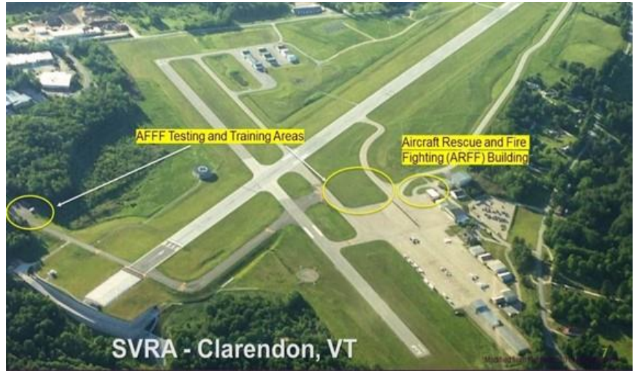
Southern Vermont Regional Airport AFFF testing and training areas.
