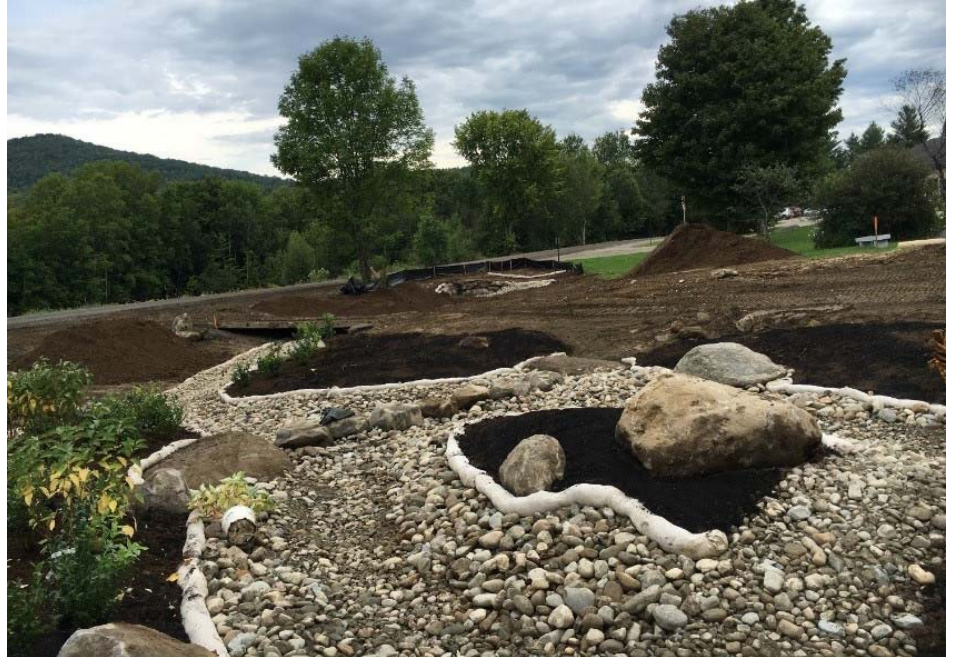
The stormwater retrofit practice installed at the school treats runoff from more than one acre of previously unmanaged impervious surface.
