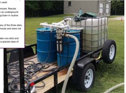
Stone Environmental designed and built a temporary water treatment system at the Vermont Fire Academy.
