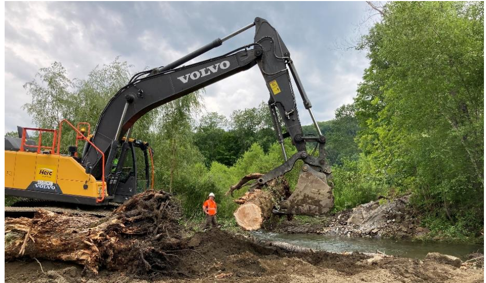
Channel construction following dam removal on Broad Brook in Guilford, VT.
