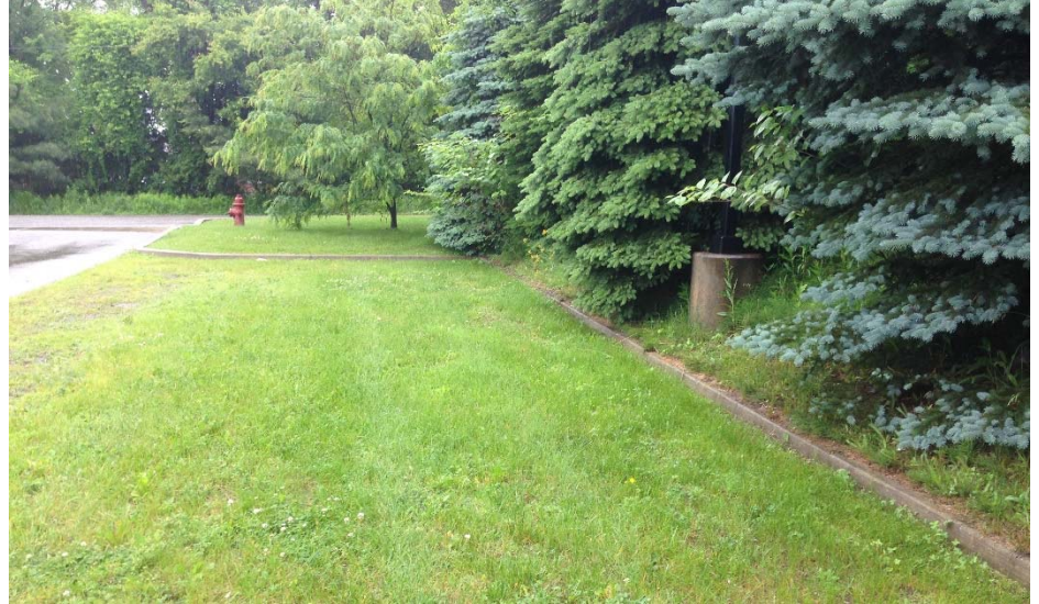
This overflow parking area surfaced with grass pavers (at Advanced Auto in South Burlington) is one example of the green stormwater infrastructure practices that may be implemented under the new LDRs.
