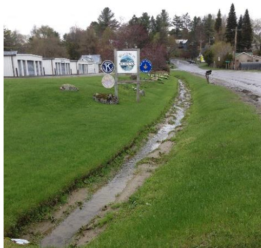
The drainage ditch along VT Route 14 in Hardwick carrying flow and runoff from a 111- acre drainage to Cooper Brook before (left) and after (right) channel and floodplain restoration improvements were completed in 2020.
