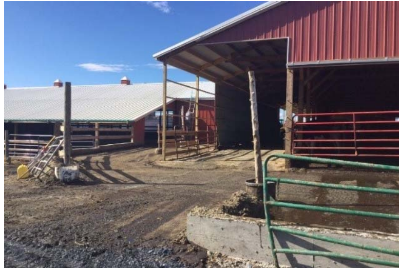
Working under contract with AAFM, the Stone team designed an earthen manure pit with concrete push-off ramp to improve manure management at this Addison County farm.
