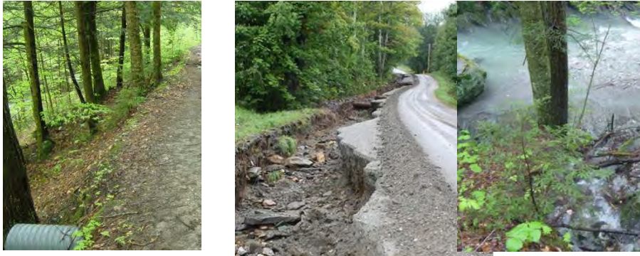
Figure 1: Evidence of water quality impacts associated with unpaved roads in Vermont's uplands: erosion of rills and gullies on impervious road surface (left panel), eroded roadside ditch resulting from channelized stormwater runoff (middle panel), direct discharge of road runoff to receiving stream from road culvert (right panel).
