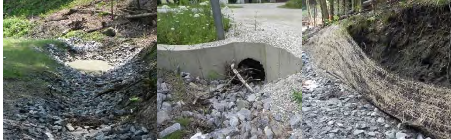
Figure 10: Examples of assessed BMPs—left: intact stone lined ditch; middle: culvert compromised by debris partly plugging inlet; right: failed BMP installation showing evidence that stone and stabilization fabric have been undermined.
