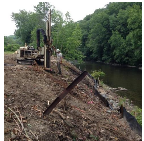
Advancing soil borings along the bank of the Black River.
