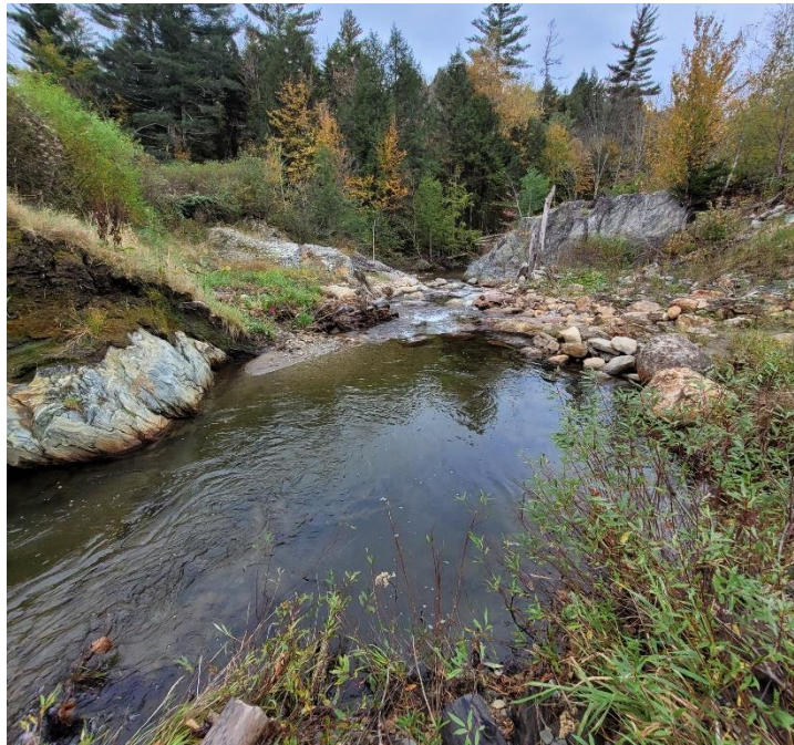
Looking downstream at the former Johnsons Mill Dam location along Bogue Branch in Bakersfield, Vermont in 2023.
