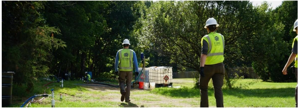
Stone staff members monitor injection procedures at the Commerce Street Superfund Site in Williston, Vermont.
