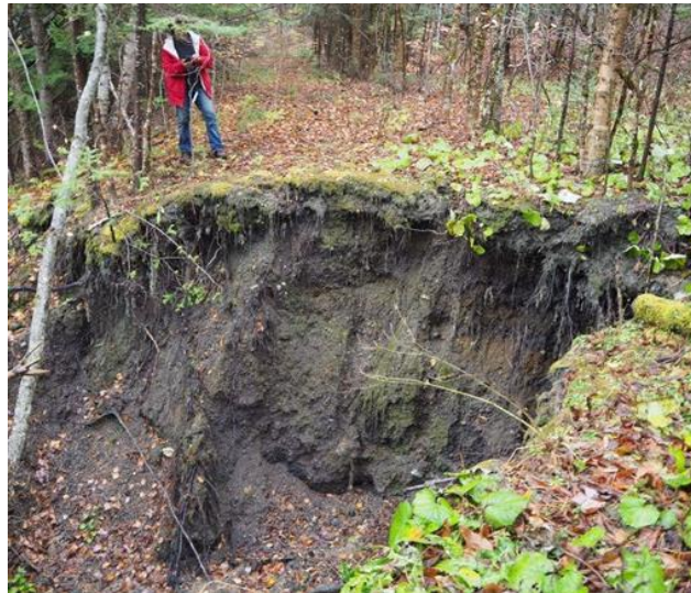
One of several headcuts across the abandoned rail bed identified during field survey (left). UAV LiDAR-derived topo contours and were loaded into a mobile field data collection app to quickly identify problem areas (right).
