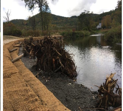
Eroding bank along meander bend of Stevens River adjacent to private property and horse farm (left); same meander bend following construction of bank stabilization measures (right).
