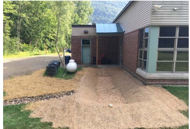
A bioretention area, shown above just after construction, captures and treats runoff from the school's rooftop.
