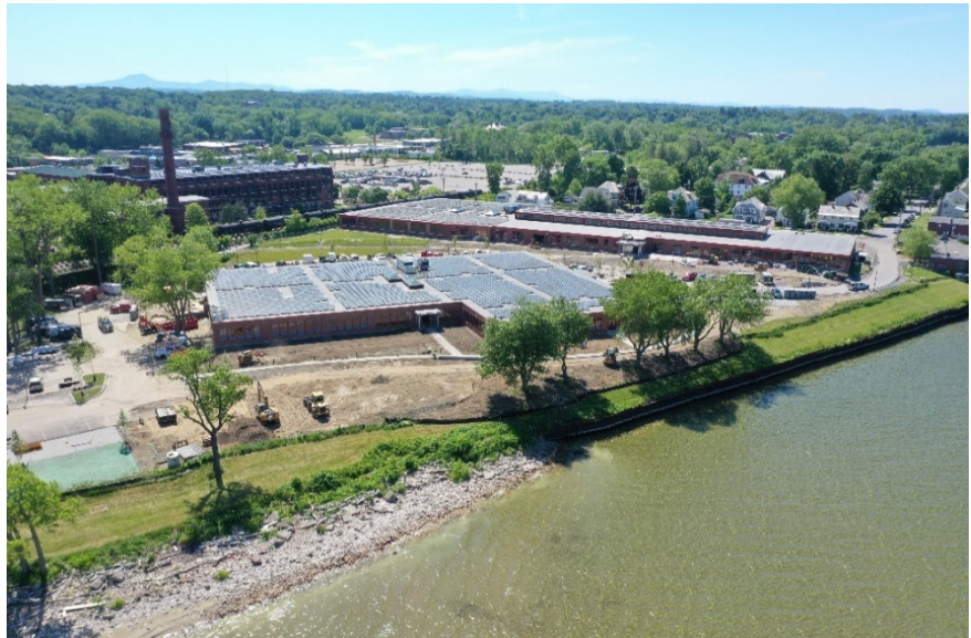
Project site seen from Lake Champlain. The rooftop of 50 Lakeside Ave. has been outfitted with solar panels.
