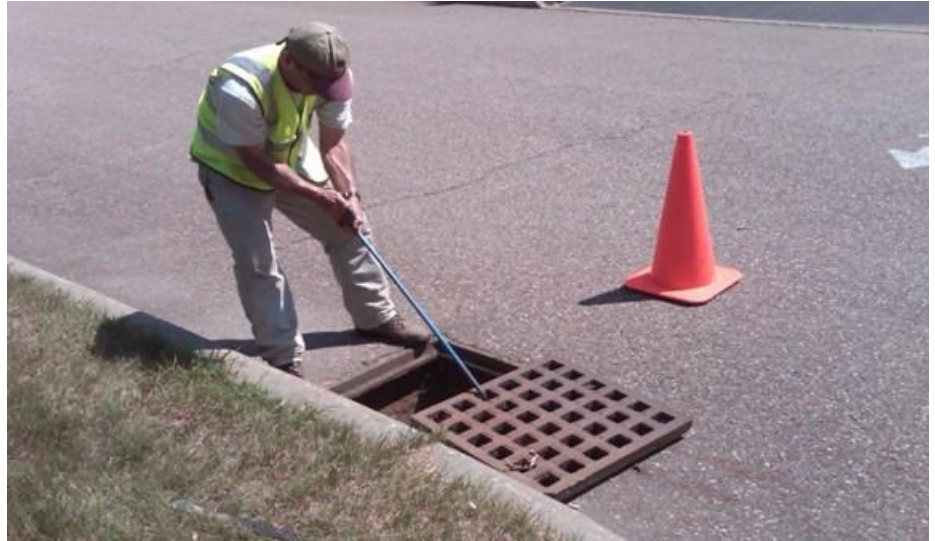
Stone field staff replacing a catch basin grate after documenting materials, dimensions, condition, and connections.
