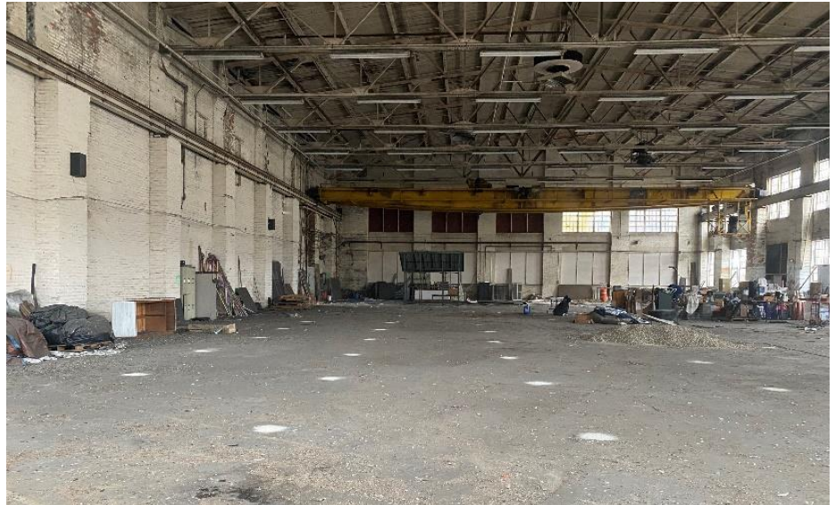
Interior of former Plant #4 foundry building.
