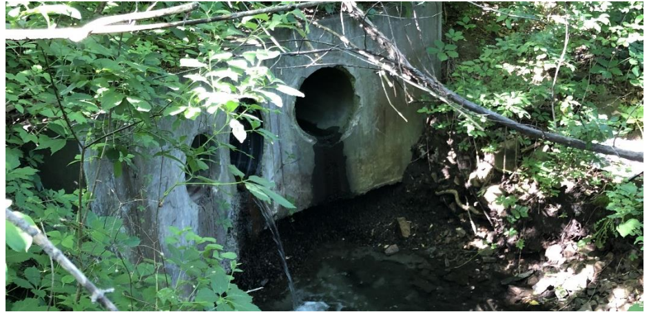
View of outfall discharge location to Centennial Brook.
