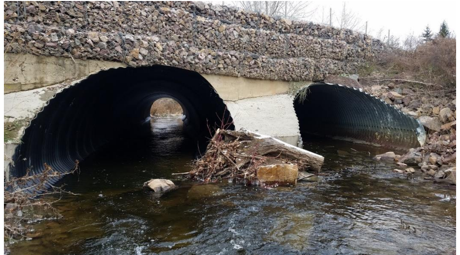
Stone documented site conditions at each culvert. Photo shows culverts at Talcott Road looking downstream.
