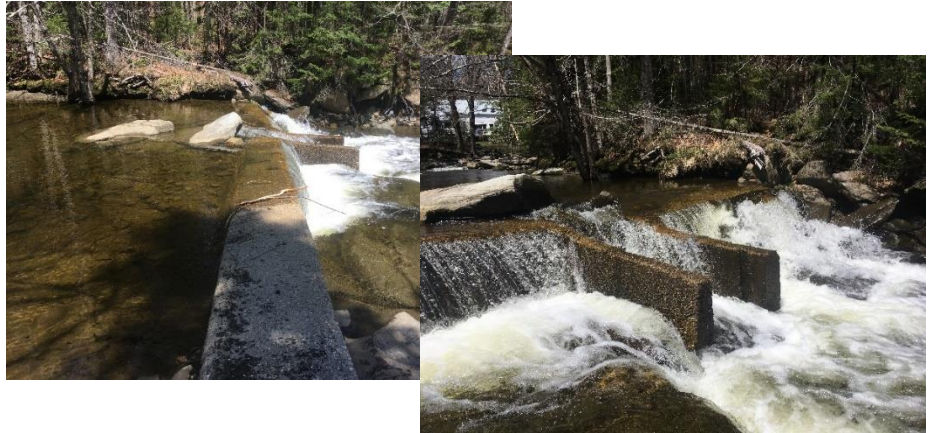
View along top of dam, looking northeast (left); View of dam and sluice, looking north (right). During a topographic survey in May 2017, Stone observed brook trout trying to unsuccessfully jump over the dam. (Source: Stone)
