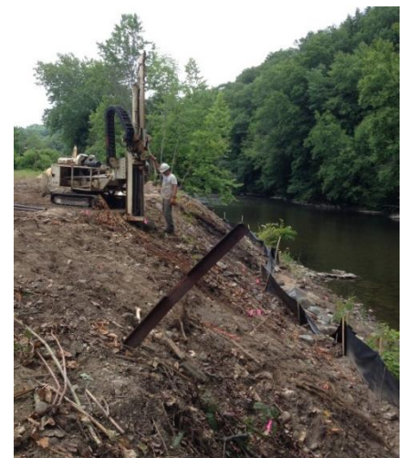
Advancing soil borings along the bank of the Black River.
