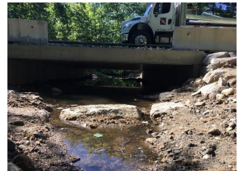
Left: Top sections of box culvert being installed following bottom section and channel bed material installation. Right: Completed channel restoration and box culvert installation, prior to final roadway improvements (paving, guardrail installation, etc.).
