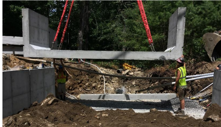
Concrete box culvert installation at Seaver Brook and Pollard Road, August 2020.
