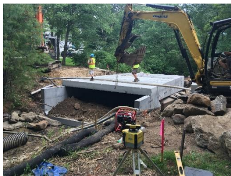
Left: Top sections of box culvert being installed following bottom section and channel bed material installation. Right: Completed channel restoration and box culvert installation, prior to final roadway improvements (paving, guardrail installation, etc.).
