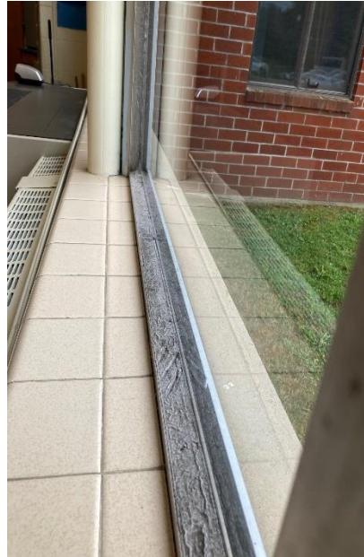
Suspected PCB-containing building materials in schools: Left – window caulk, Upper Right – covebase adhesive and green paint, Lower Right – Fluorescent light ballast and cover
