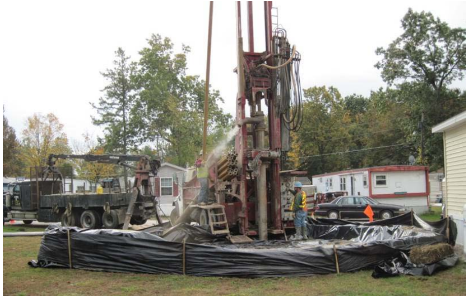
Bedrock Drilling in Support of Savage Municipal Water Supply Superfund Site – Operable Unit 3
