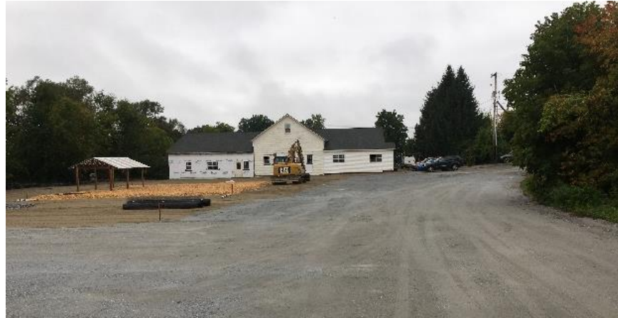
Engineered barrier installed site wide.
