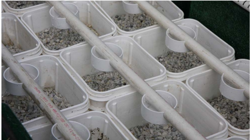
A packed-bed media filter for phosphorus removal from onsite wastewater, utilizing water treatment residuals and designed based on Stone's research and specifications, in action.
